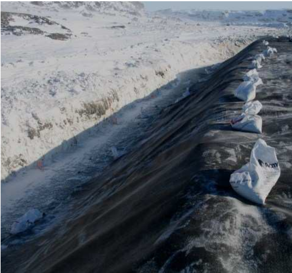
Photo 8: Geotextile placed Sta 2+95 to Sta 3+30
