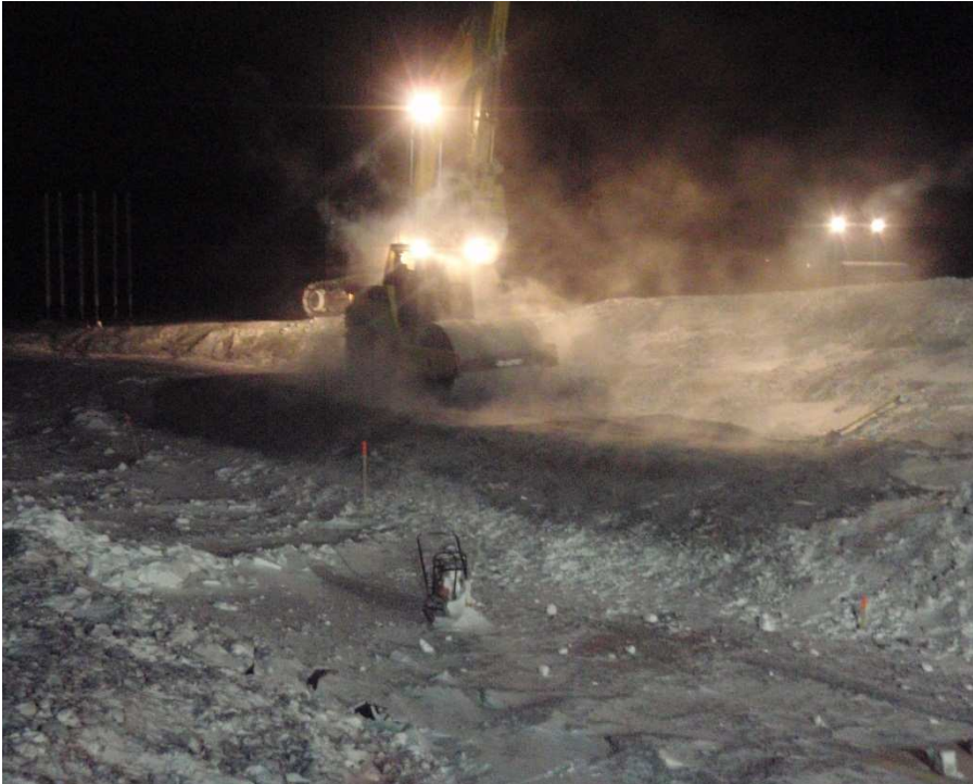
Photo 13: Excavator and packer working on underbuilt SSE corner
