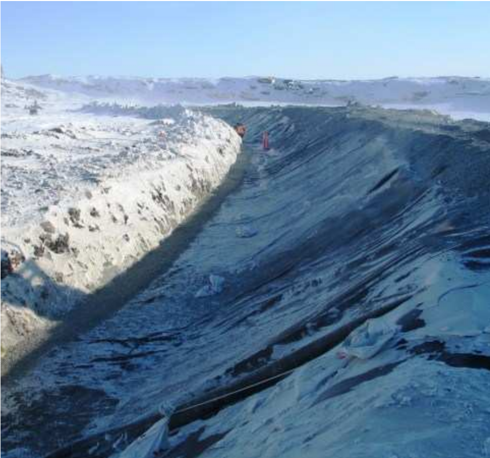
Photo 9: Bentonite placed over liner Sta 3+30 to Sta 3+90
