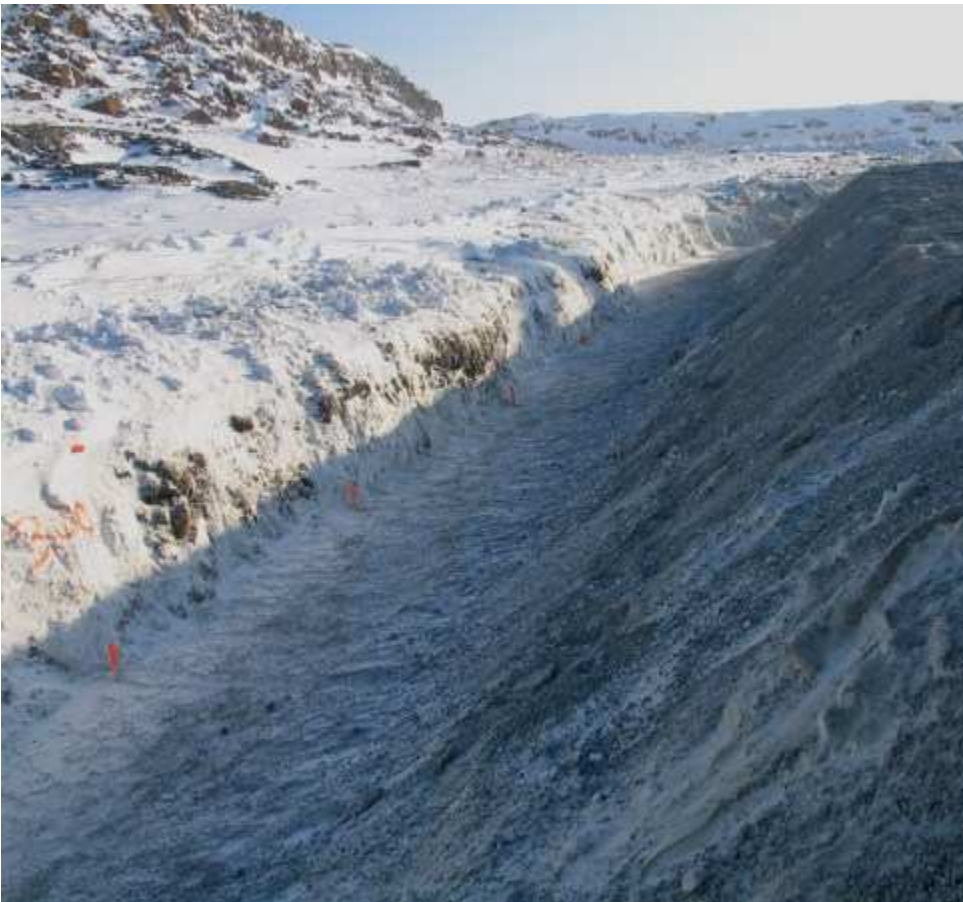
Photo 7: Trench cleaned Sta 2+95 to Sta 3+30
