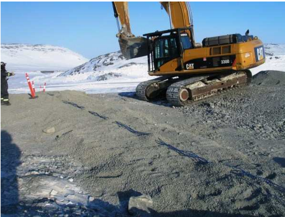
Photo 5: Multi bead cluster laid out at Sta 0+60
