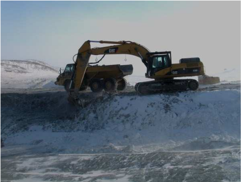
Photo 4: Excavating upstream side to top of separation material.
