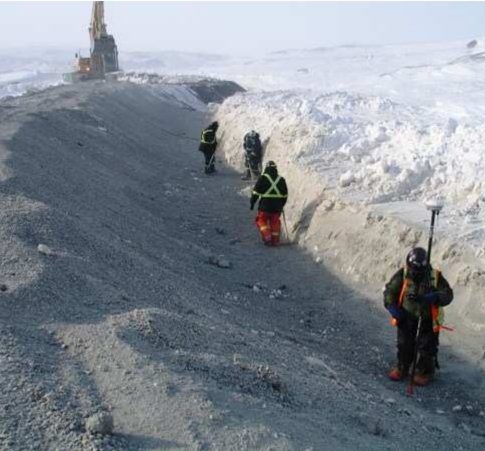
Photo 10: ¾ in crush placed over liner Sta. 3+30 to 3+90
